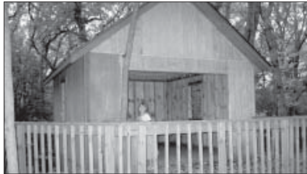
Science teacher Pat Arndt's daughter looks out over the deck of the recently constructed Lynn Seward Education Center located in the school forest near the Mascoutin Golf Course on land donated by the children of Berlin physician Dr. Lynn Seward and his wife Gladys.
